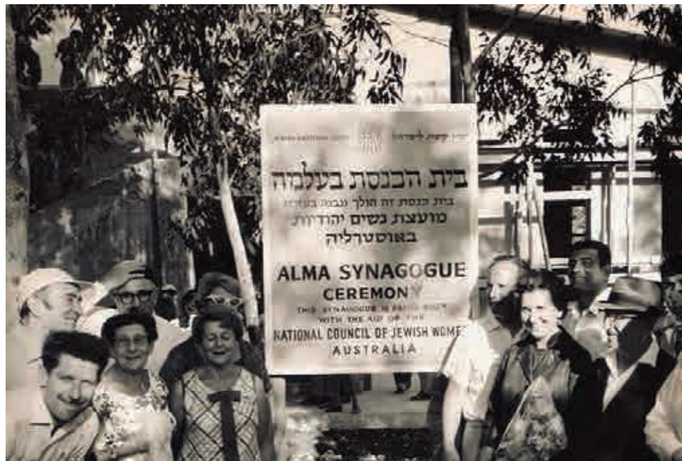
Laying of the foundation stone for the synagogue in Alma settlement Israel
